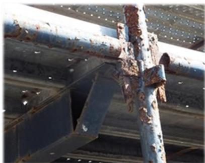
**Figure 9** Severe corrosion on critical scaffolding components
