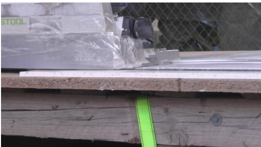
Figure 5: Stone slab sitting on chipboard sheet used as a backer-board.
