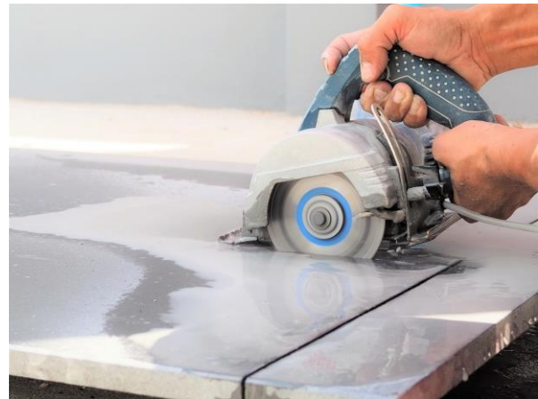
Figure 1: Water suppressed stone saw.
