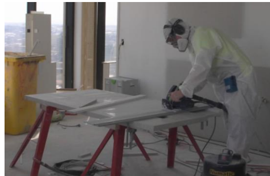
Figure 6: Worker cutting a stone benchtop in a high rise.
