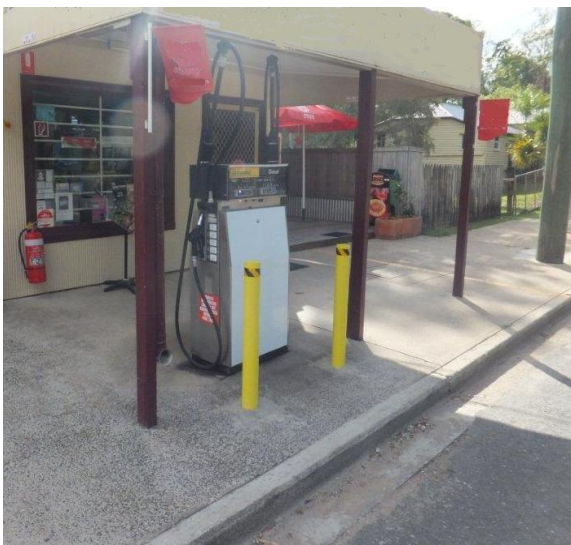
Figure 1: A typical kerbside fuel dispenser.
