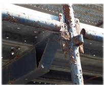
Figure 9 Severe corrosion on critical scaffolding components
