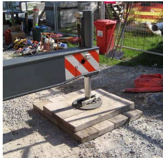
Photo 3: Example of good outrigger support
