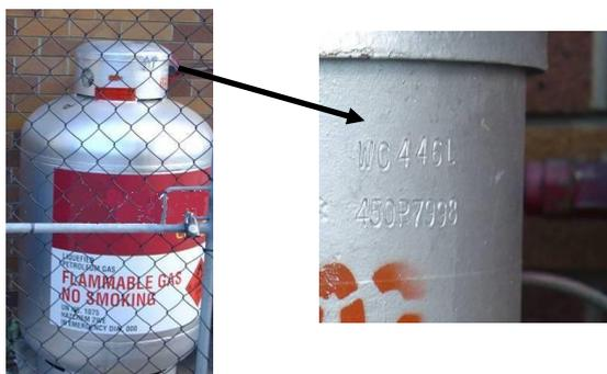
**Figure 13.** Gas cylinder and a close-up view showing WC value.
