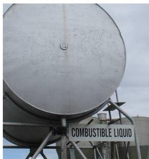
Figure 6: Combustible liquid placard.
