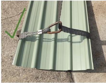
Figure 4: A steel webbing sling being used to lift roof sheeting – edges will not damage this type of sling
