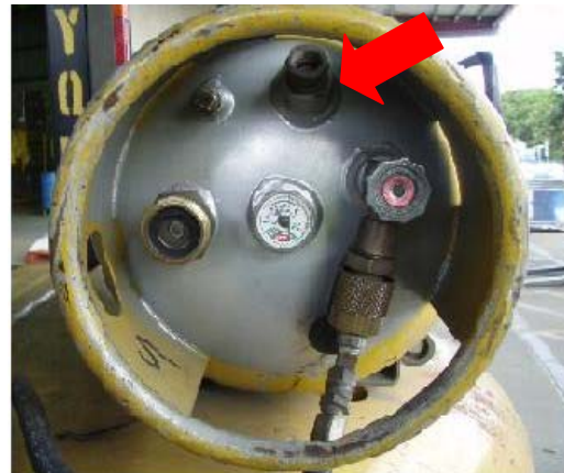
Image: LPG cylinder on a forklift showing the relief valve located in the correct position at the top.
