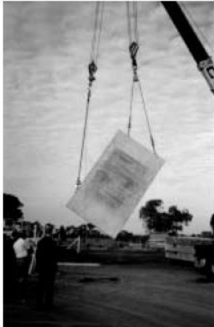
Figure 16 Rotation of a precast element – not to be lifted over workers
