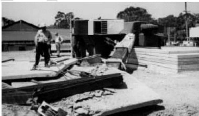
Figure 8 Rubber tyred pick and carry crane overturned
