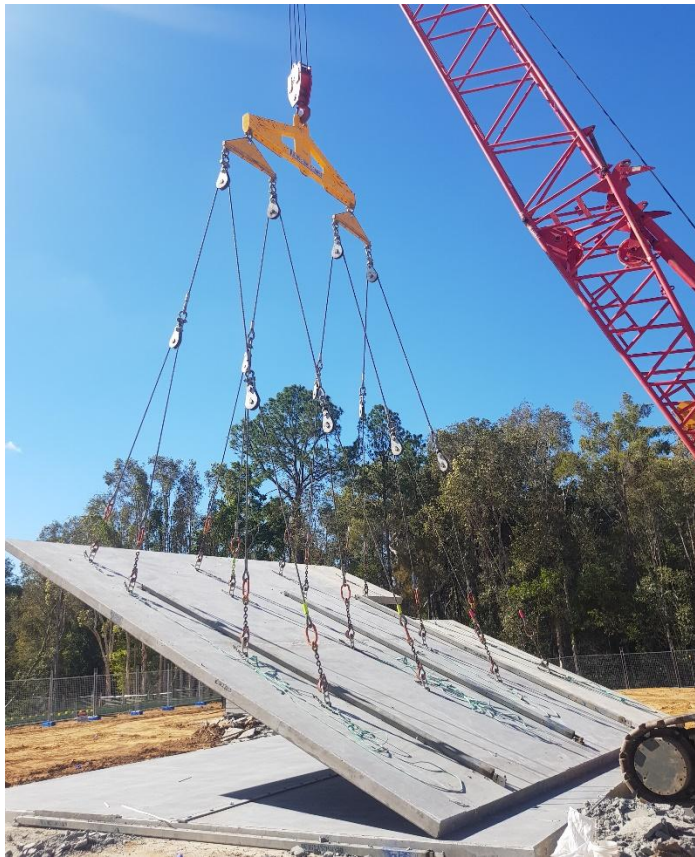
Figure 13 Tilt-up panel being lifted off casting stack
