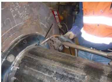
After: welding gun supported by fully adjustable stand
