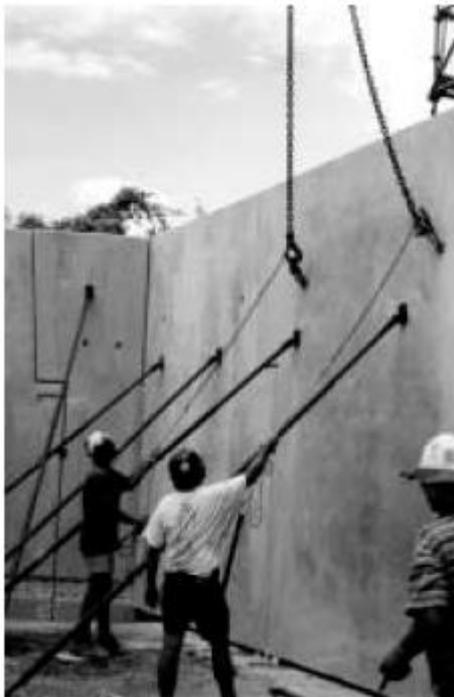
*Diagram 9 – Lifting clutch release lines*
