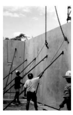
Diagram 9 - Lifting clutch release lines
