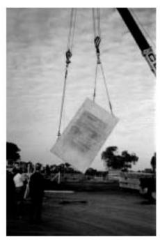
Diagram 11 - Rotation of a pre-cast panel
