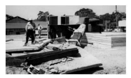
Diagram 7 - Rubber tyred pick and carry crane overturned
