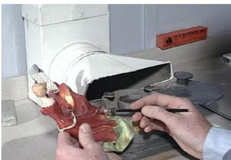
Figure 13A: Fixed exterior hood (HSE UK)
