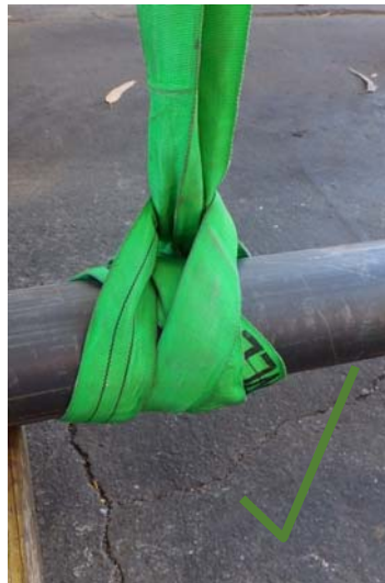
Figure 6: Round webbing sling with double wrap choke around steel pipe – large radius so sling protection not required
