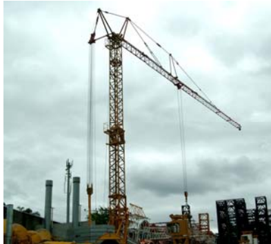
Figure 13 – Self-erecting tower crane
