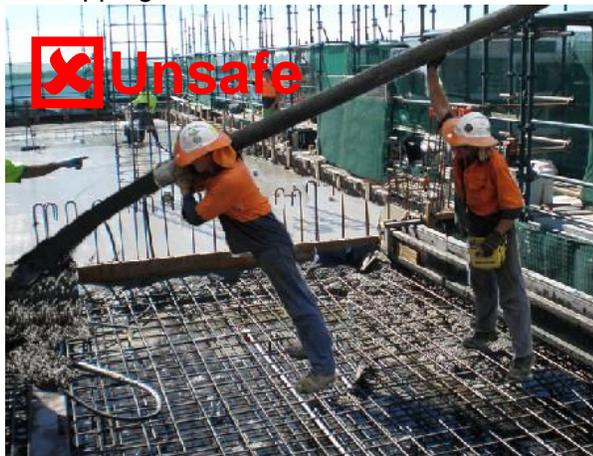
Figure 4 – Workers stretching hose for additional reach. This is an unsafe work practice
