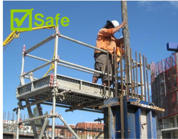
Figure 5 – Pouring concrete into column form.
