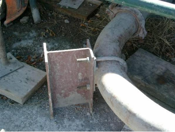
*Figure 2. One method of anchoring pipe.*
