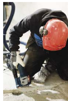
Figure 13B: Cutting concrete with HVLV extracted device (Source: Dustcontrol UK)
