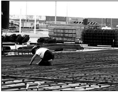
Steel fixing
