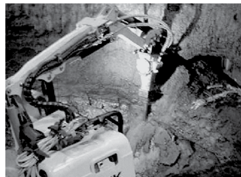
Figure 2: Remote controlled excavator
