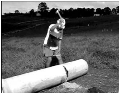
Cutting concrete pipe with hammer
