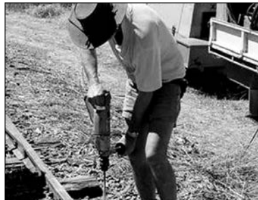
Operating power drill
