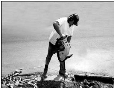
Operating petrol-powered jack hammer
