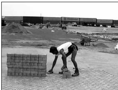
Laying paving blocks
